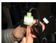
Figure 46: Pressostat de pression maximale.
