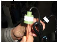
Figure 41: Pressostat de pression maximale.
